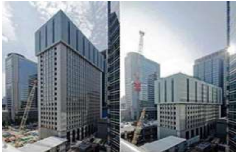
Fig. 2. Skyscraper demolition using the TEcoRep technology [13].
