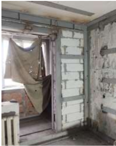
Fig. 16 Restoration of wall panel No. 1.
