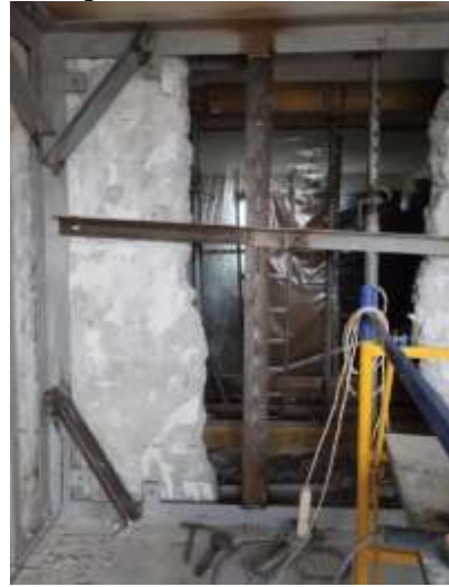
Fig. 17 Dismantling of wall panel No. 3.
