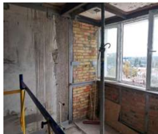
Fig. 15 Dismantled wall panel No. 1.
