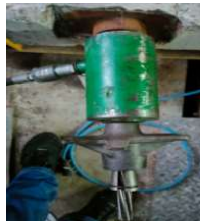
Fig. 6 Creating tension using a jack.
