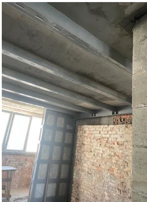
Fig. 14 Reinforcement of the floor slab after a fire by adding steel beams. Photo by V. Nuzhnyi
