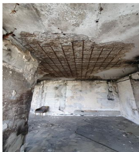
Fig. 11 Effects of fire on floor slab. Photo by V. Nuzhnyi
