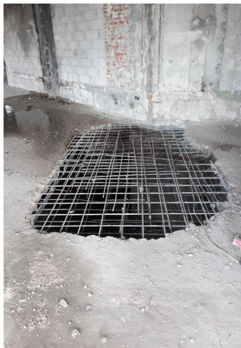
Fig. 13. Cleared area of the ceiling after the fire, shown in Fig. 12. View from the upper floor. Photo by V. Nuzhnyi
