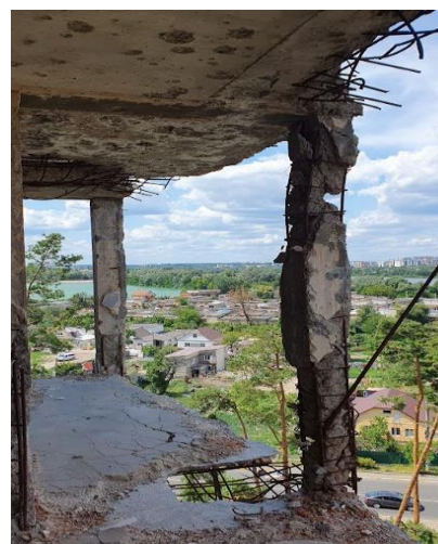
Fig. 6 Damage to the frame slab and columns. Photo by V. Nuzhnyi
