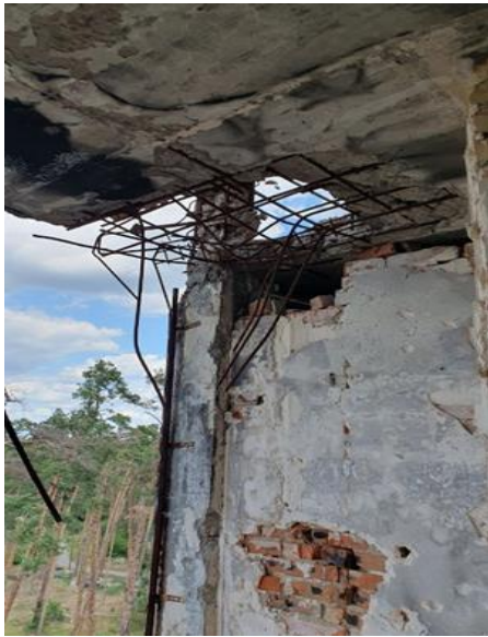
Fig. 7 Damage to the frame plate from Fig. 6, bottom view. Photo by V. Nuzhnyi
