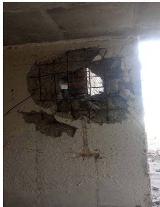
Fig. 9 Through-hole damage to the pylon. Photo by V. Nuzhnyi
