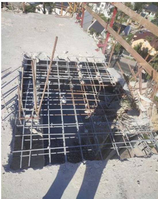
Fig. 8 Cleared impact zone from Figs. 6 and 7, which nearly corresponds to the dimensions of a structural bay. Photo by V. Nuzhnyi
