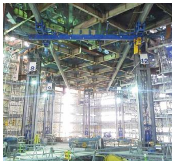
Fig. 2 The utilization of the existing roof structure (Source: Taisei Corporation)
