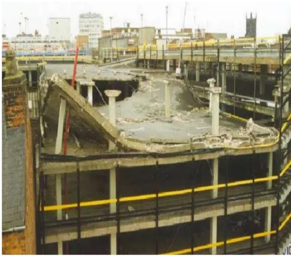
Fig.1 Collapsed 4th floor slab at Pipers Car Park, Wolverhampton on 25/03/1997 Photo by Wood J. G.M [1]
