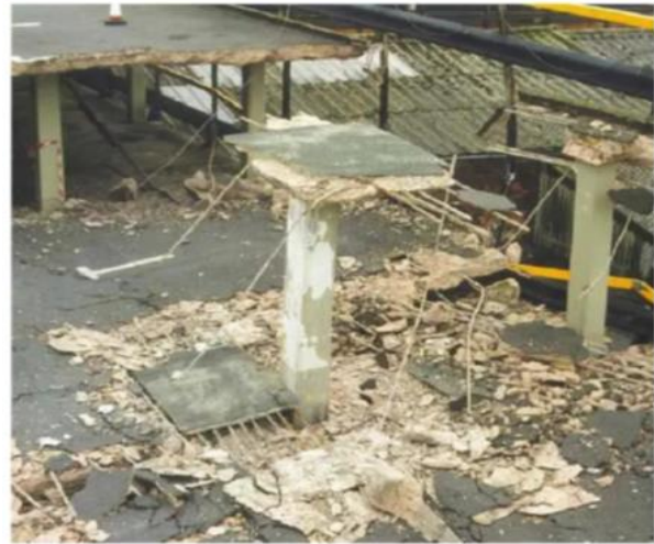
Fig.1 Collapsed 4th floor slab at Pipers Car Park, Wolverhampton on 25/03/1997 Photo by Wood J. G.M [1]
