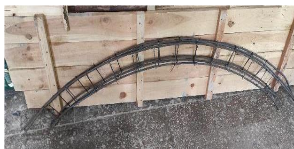
Fig. 2. General view of the manufactured frame.
