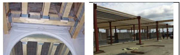
Fig. 9. The use of metal-timber beams during reconstruction
